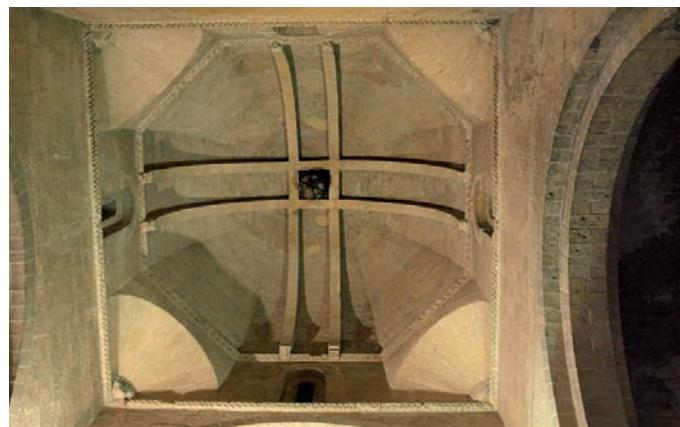
The arms of the crossing are covered with half barrel vaults and the dome of the crossing is placed on conical vaults of caliphal architecture.
